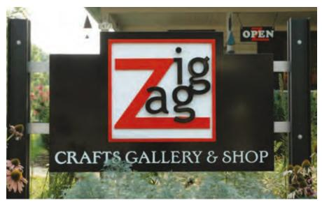
Carved Extira backer panel with raised/applied HDU logo panel. Posts are double steel c-channel with exposed stainless steel hardware for fun.
